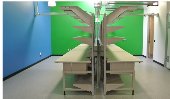
Plug-play power and data runs from the ceiling for easy reconfiguration in this technology lab.
